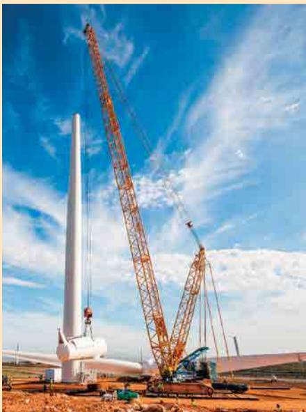
A Siemens turbine being assembled at the Jeffreys Bay Wind Farm. The project has been operational since mid-2014.
