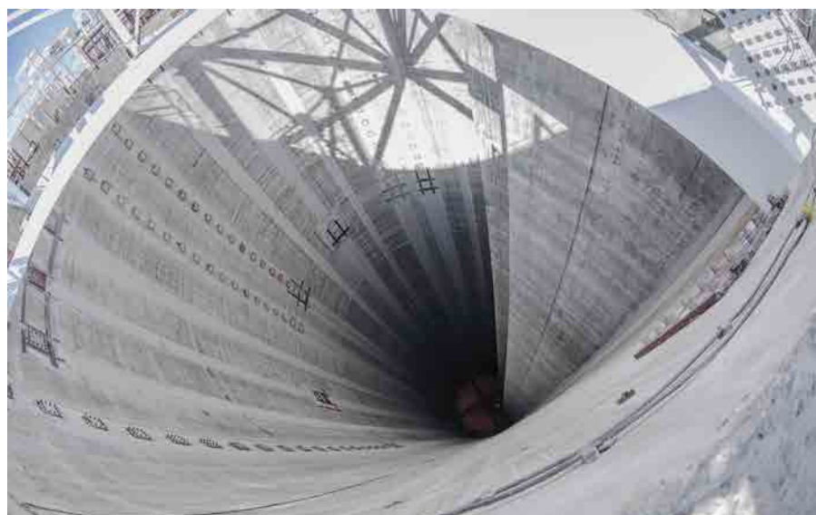
A shot down the tower from the top. It doubles as a cooling tower so at the top there is a strong wind blowing upwards as the hot water at the bottom heats the air. The tower is equivalent in height to a 50-storey building. Photo: Christy Strever
