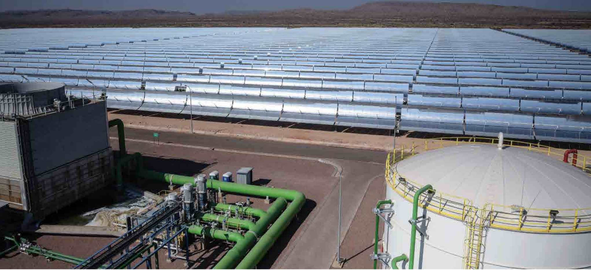
250 hectares are covered in parabolic trough mirrors, all curved to focus the sun's rays on a central heat collector. Photo: Christy Strever
